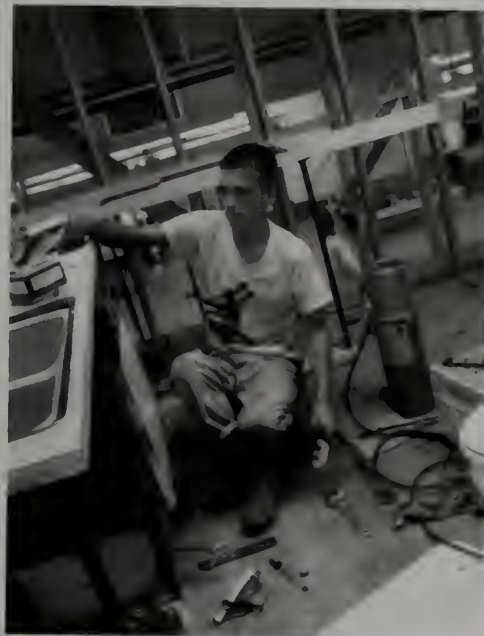
DJ Deptula installs a kitchen sink in the Plumbing Shop.
